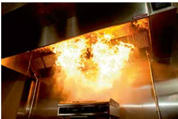
Figure 3: A fire within the duct can ignite combustible materials outside of the duct, spreading the fire in the building.
