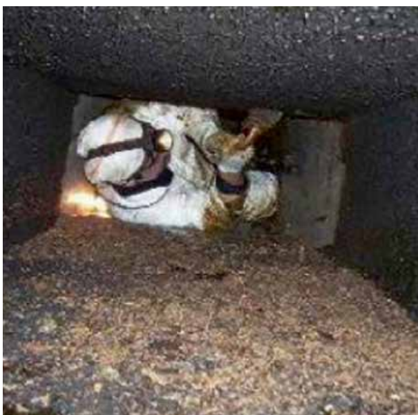
Figure 19: Checking and cleaning ductwork.
