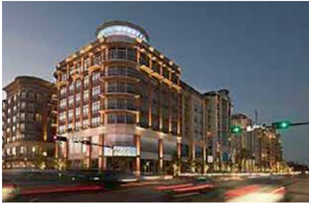
Figure 11: Multi-tenant mixed-use building.
