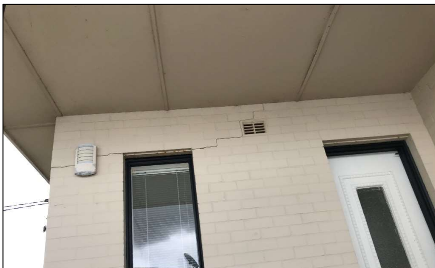
Photograph 4: Cracking observed in the external wall.
