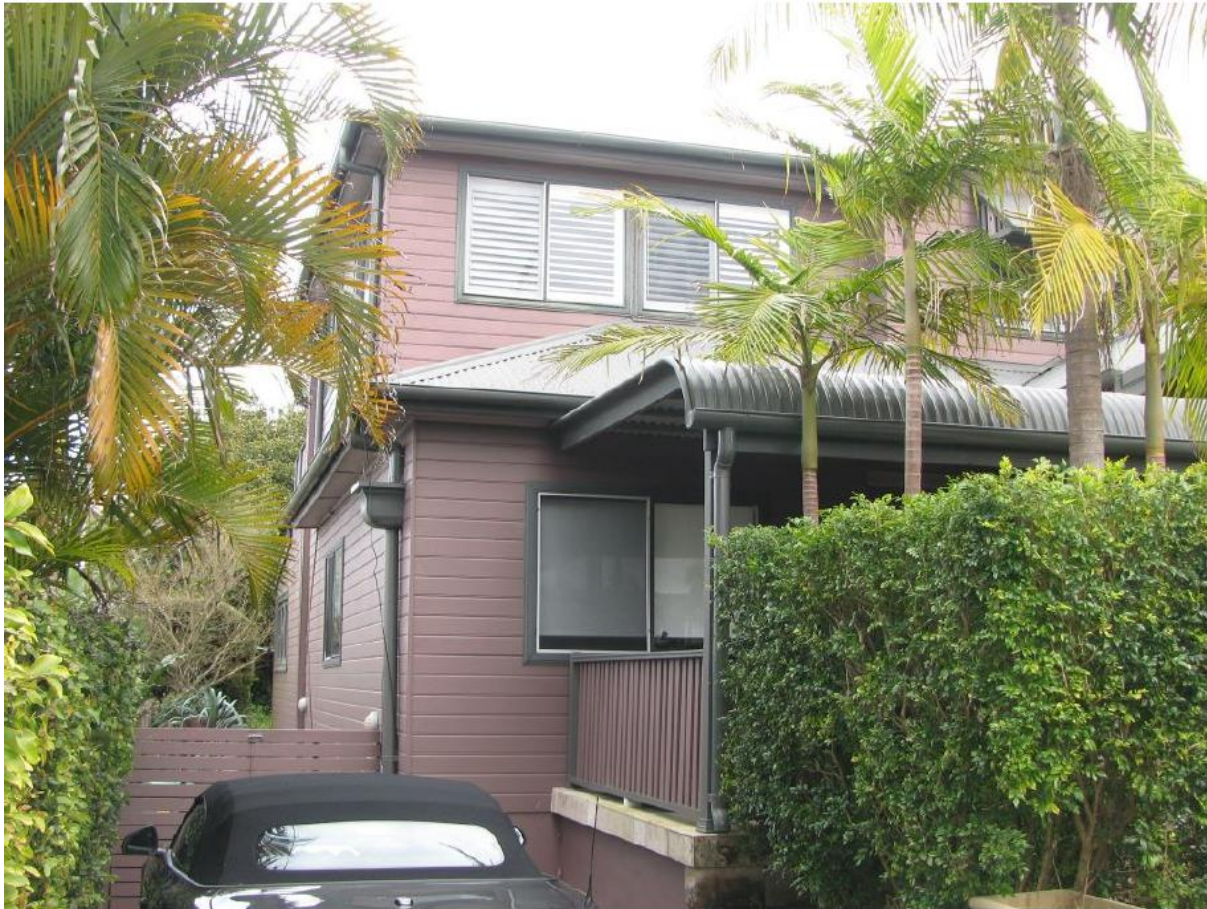
Figure 2: Street view of subject site
