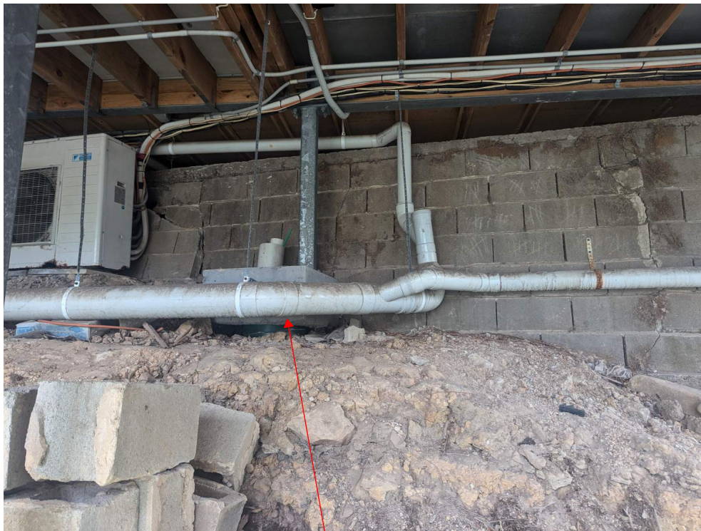
Deformed concrete block wall below suspended deck with exposed pile cap
