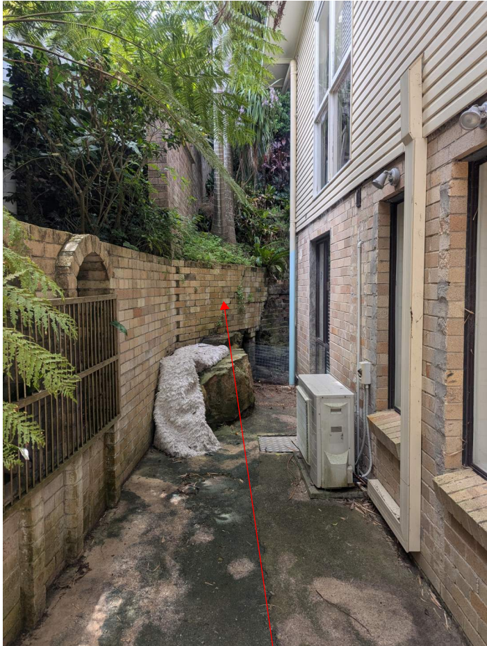
Boundary wall with No.36 and tilting section of wall
