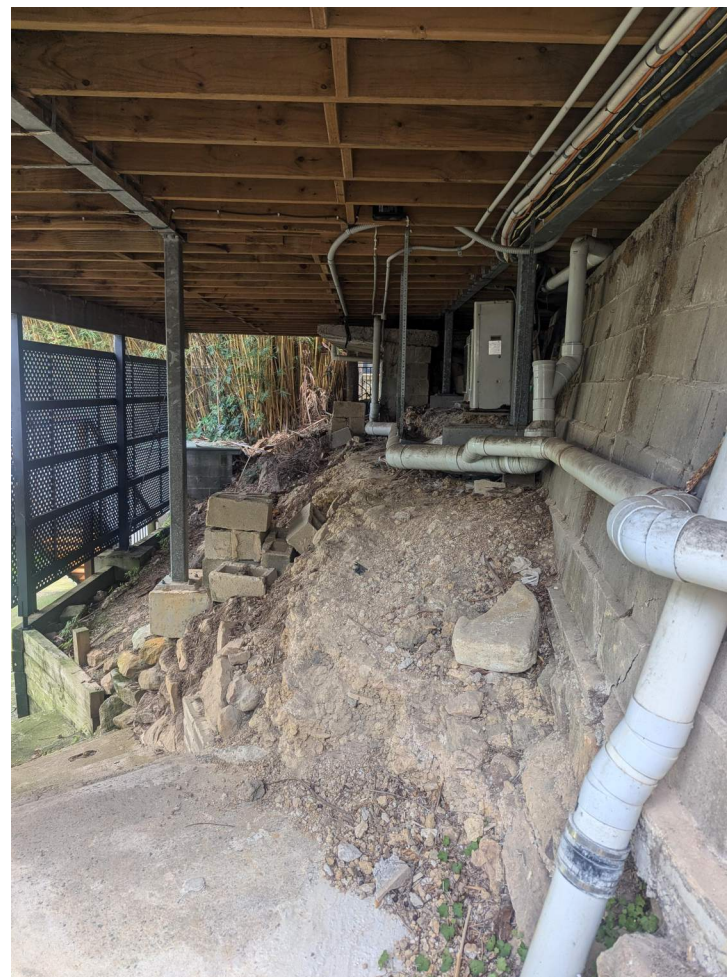
Loose fill/colluvial soils below suspended deck
