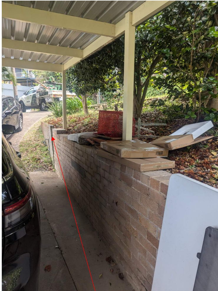
Tilting wall upslope of driveway
