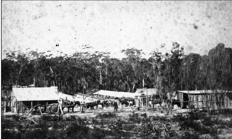
Plate 2 Brick manufacturing within the project area c.1905 (Warringah Council Library)
