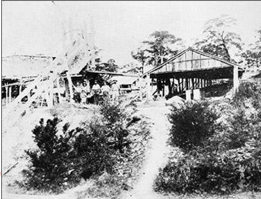
Figure 12: Hews brickworks, Frenchs Forest, c. 1905 (Source: Northern Beaches Council Library).
