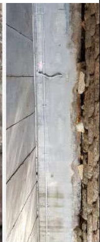
Photo No: 27 Ab Evidence of possible settlement
