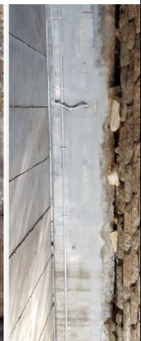
Photo No: 27 Ab Evidence of possible settlement
