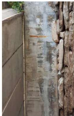
Photo No: 26 Abutment 2 Evidence of corrosion staining under unit 28.
