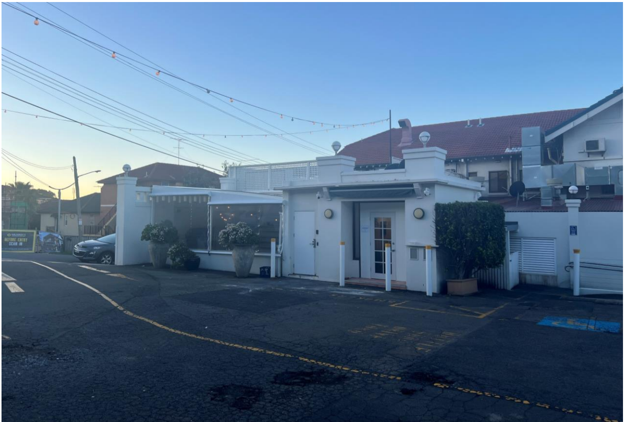
Figure 6: The Harbord Hotel as seen from the carpark
