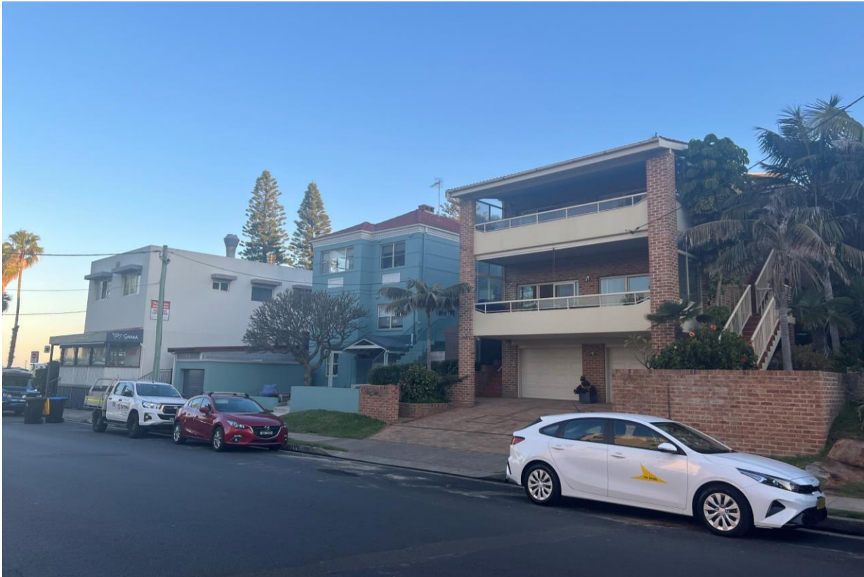
Figure 18: 33 Moore Road (right), 35 Moore Road (centre) and 37 Moore Road (left)
