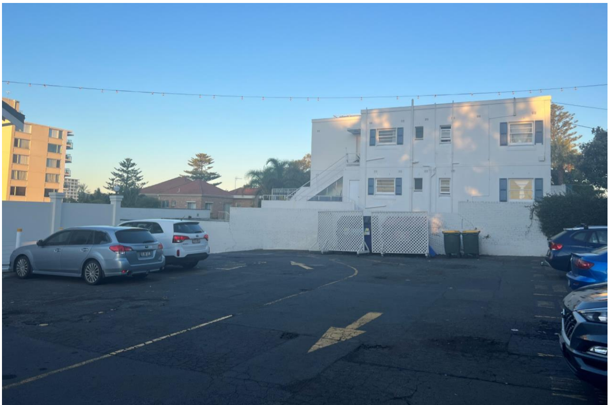
Figure 8: The rear carpark and the residential flat building at 64 Undercliffe Road
