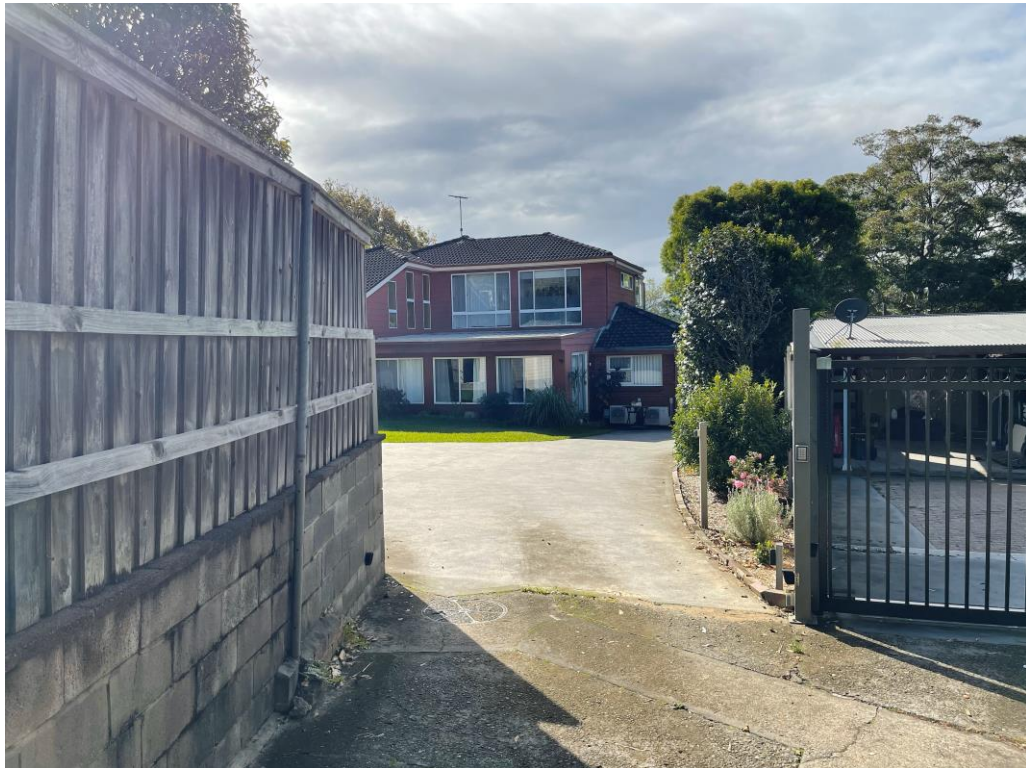
Fig 3: View of the subject dwelling, looking north from the access driveway
