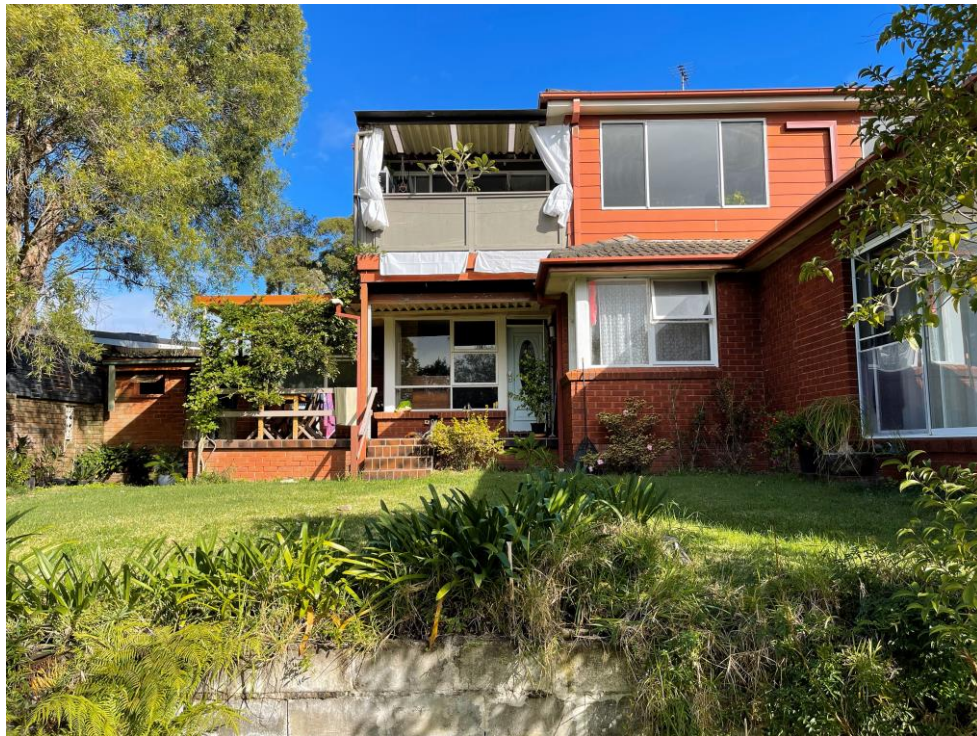
Fig 5: View of the rear elevation and location of proposed terrace extension at the ground floor level, looking south
