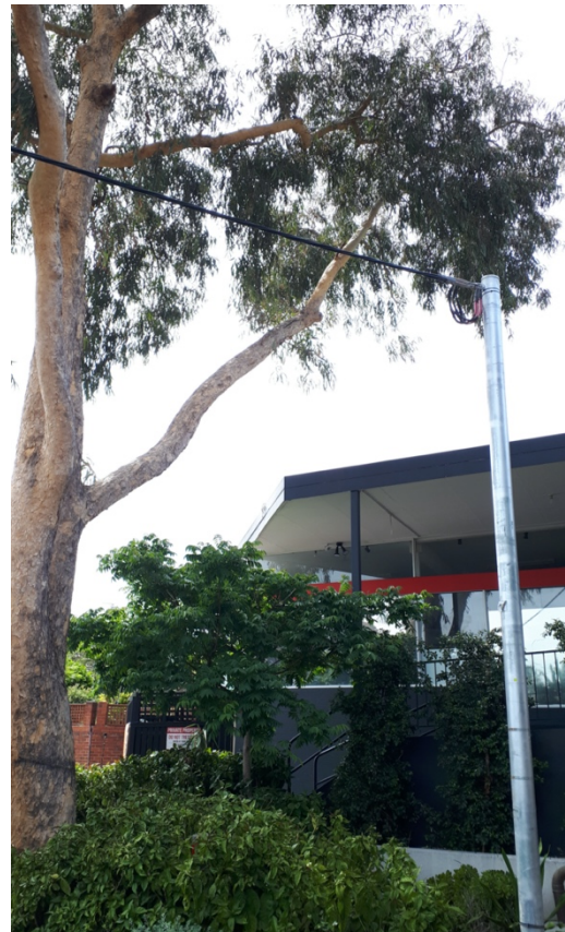
Photo 3: Looking East: Branch positioning above building.
