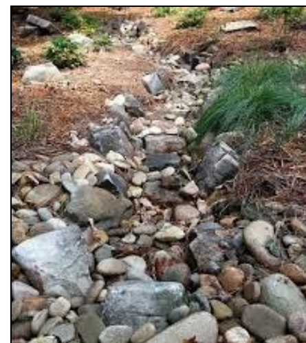
Plate 3 – Low Flow Channel (Australian Wetland Consulting, 2018)
