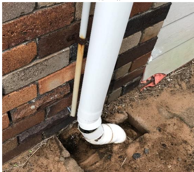
Photograph 4: Fault opening in PVC stormwater down pipe along southern external wall of site house, facing north east
