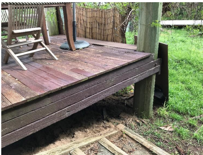
Photograph 3: Timber deck within rear of site, with rotation/rotting of timber planks and minor settlement evident, facing south west
