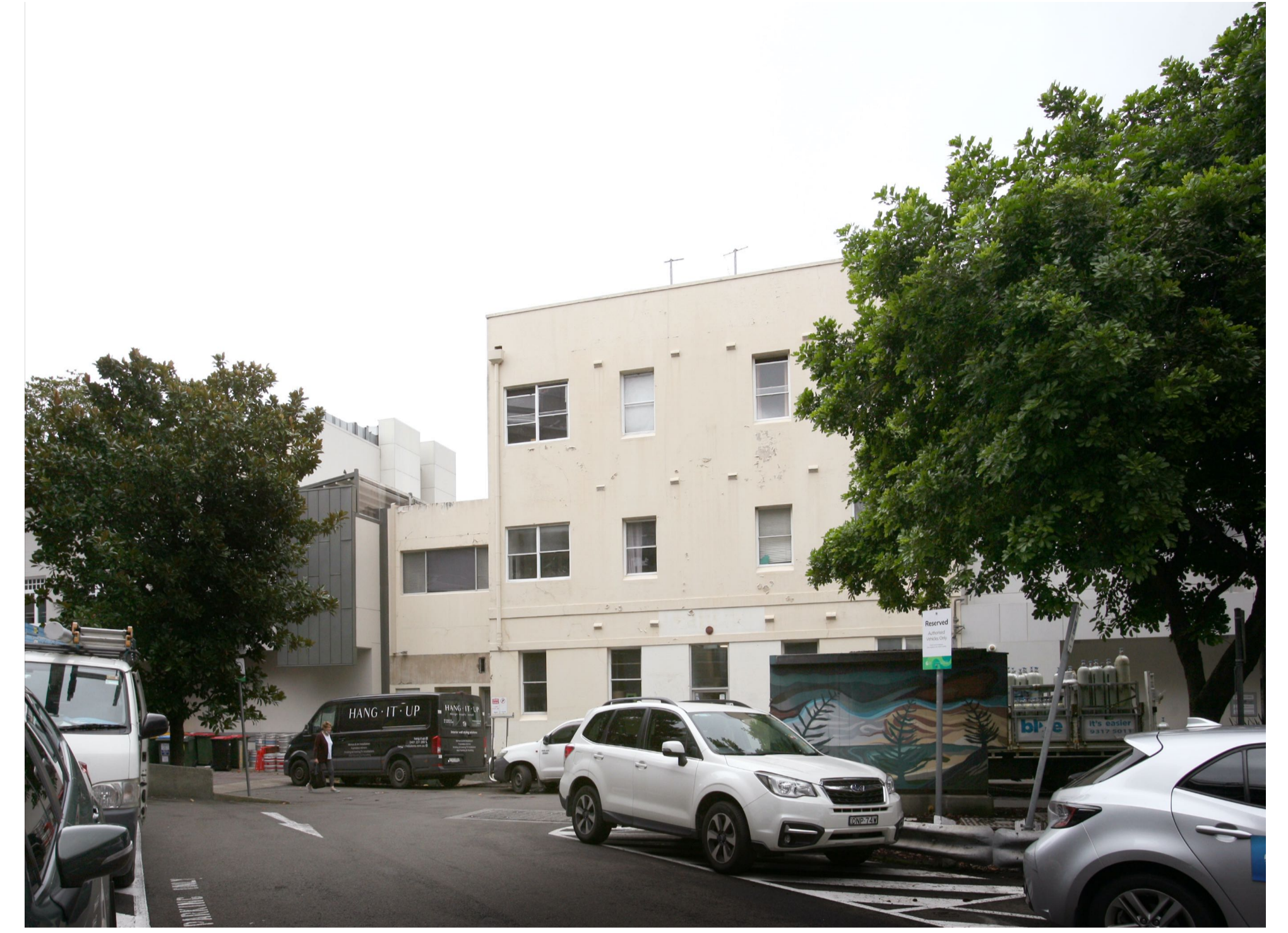
EXISTING: VIEW LOOKING FROM MARKET LANE
