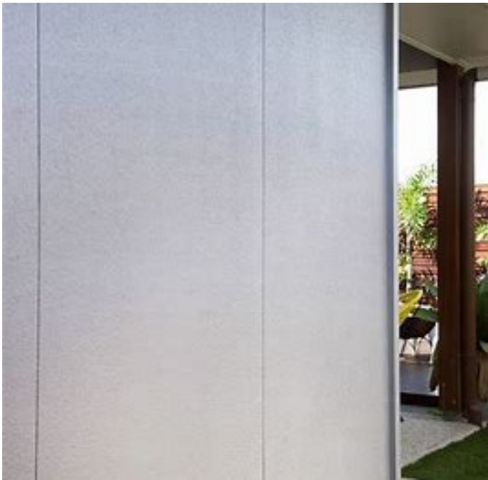
F1 FC SHEETING TO REAR UPPER LEVEL(MIN BAL RATING 40)
