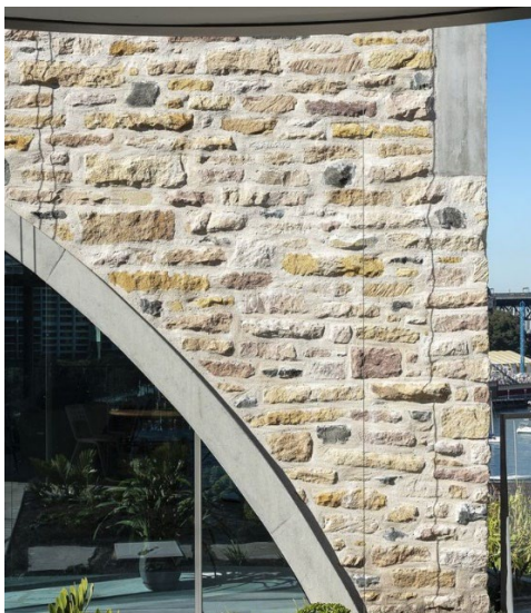
Stone Walls: Irregular Sandstone walls.
