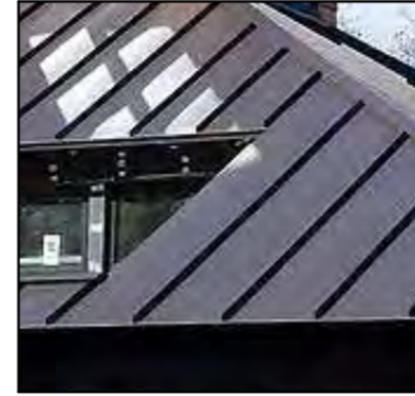
3 - SHEET METAL ROOF: COLOUR TBC BY CLIENT
