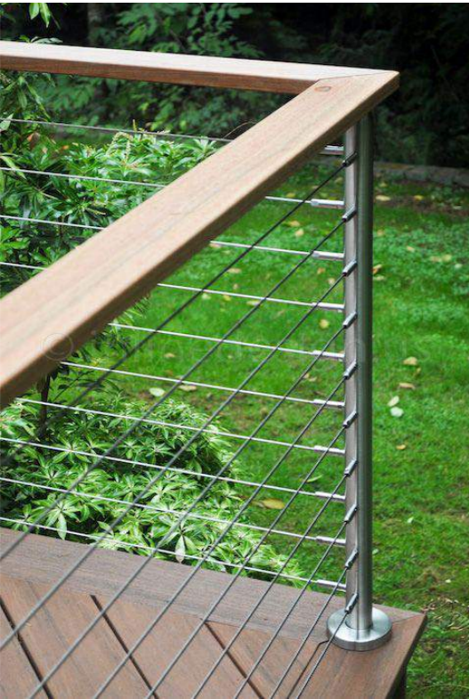
WIRE BALUSTRADE WITH TIMBER HANDRAIL
