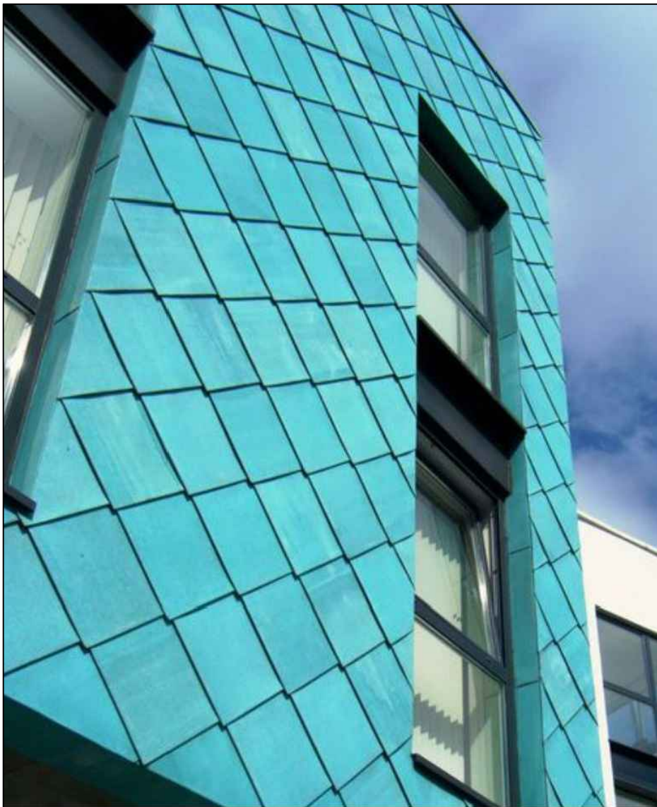
proposed diamond shaped shingle 'scales' patterned cladding. Colour proposed is Prefa '46 patina green' (natural colour) sample chip here
