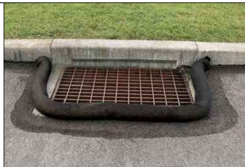
Sediment control sock to stwtr drains
