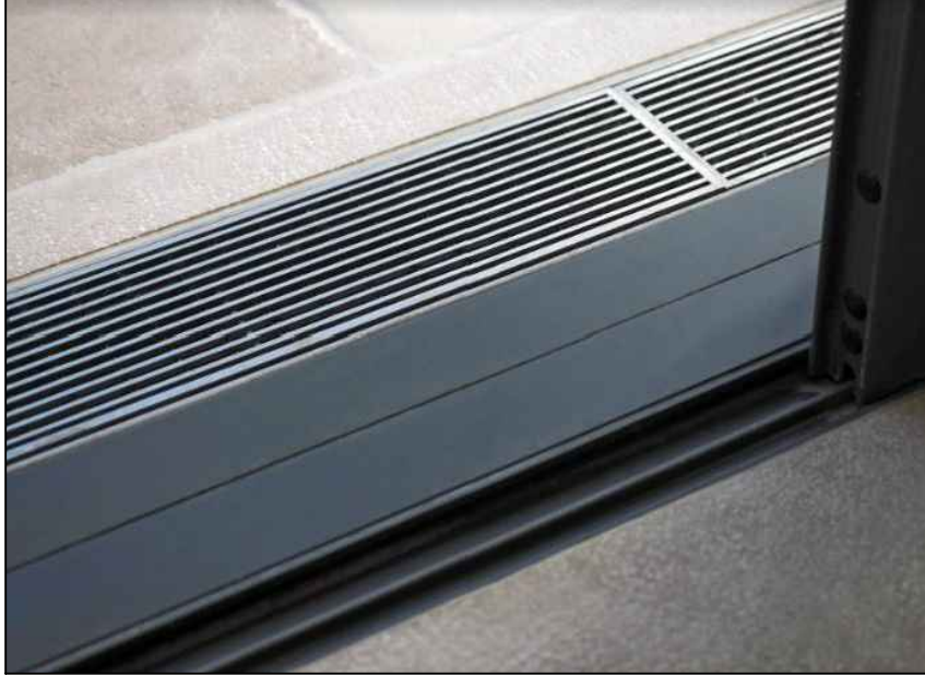
example of stainless steel slot drain to front of stacking sliders b/w new enclosed room and open balcony
