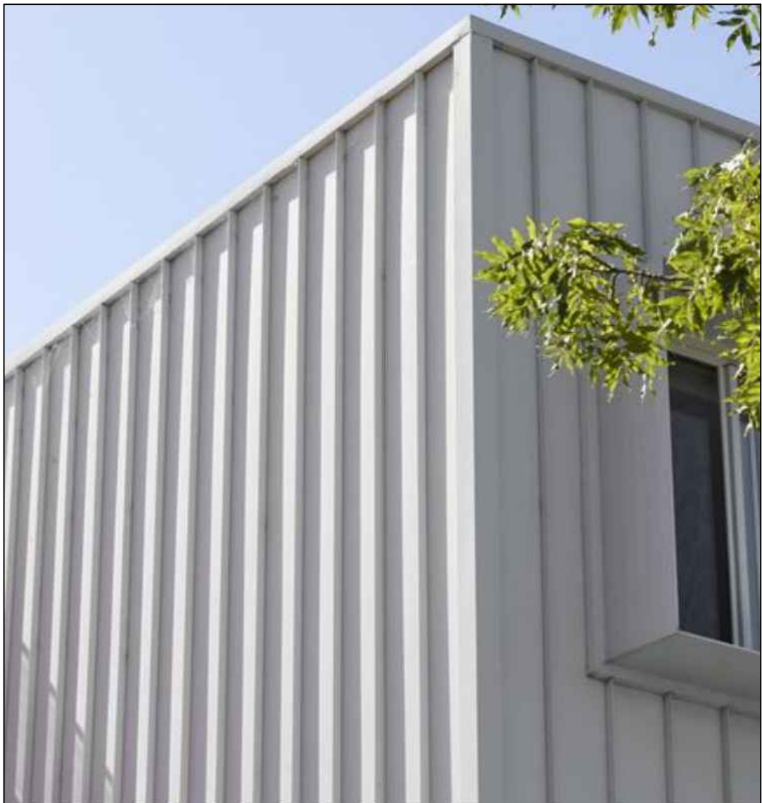
proposed PREFA aluminium metal raised seam cladding in off-white Prefa White P.10 colour
