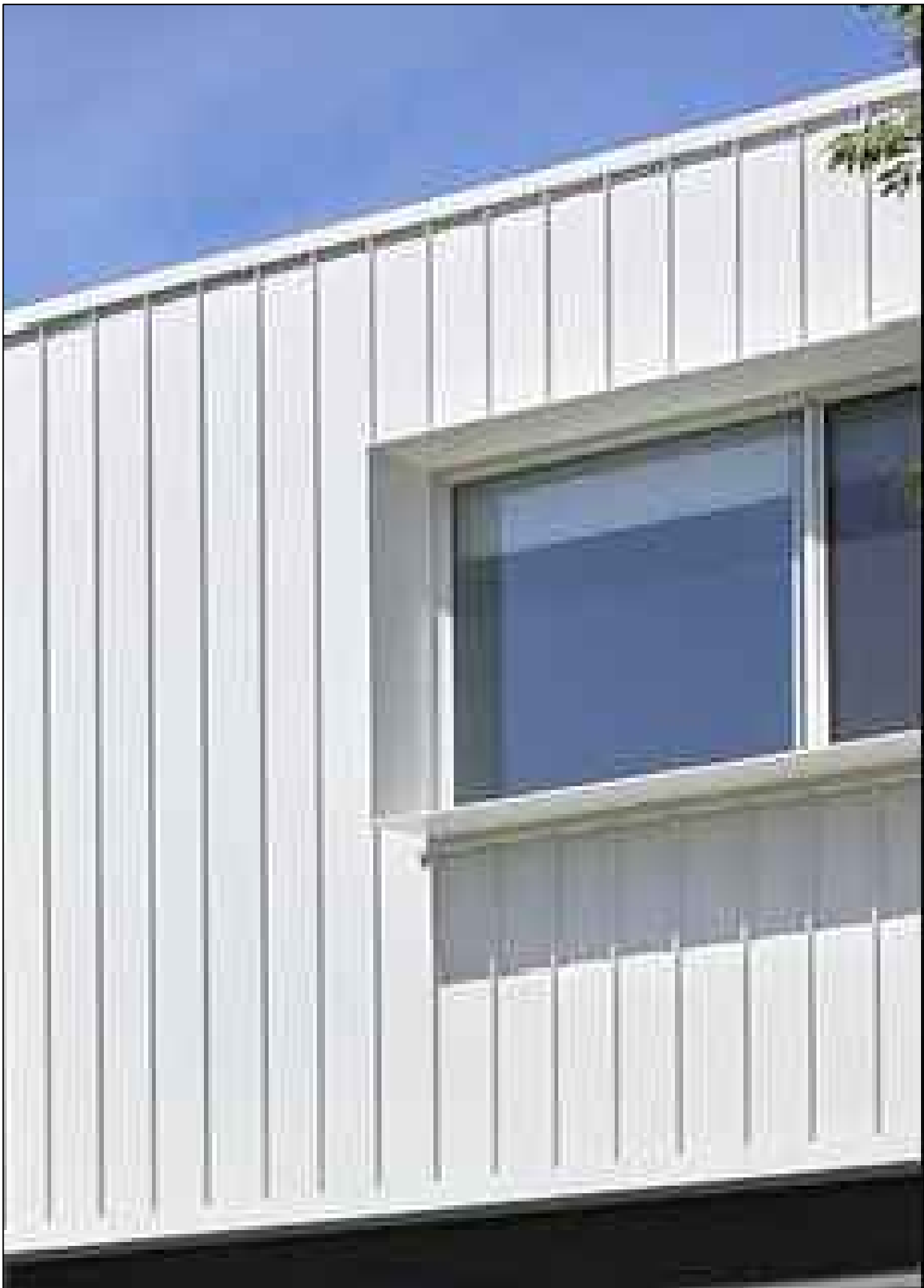
proposed raised seam PREFA aluminium metal cladding in Prefa White P.10 colour
