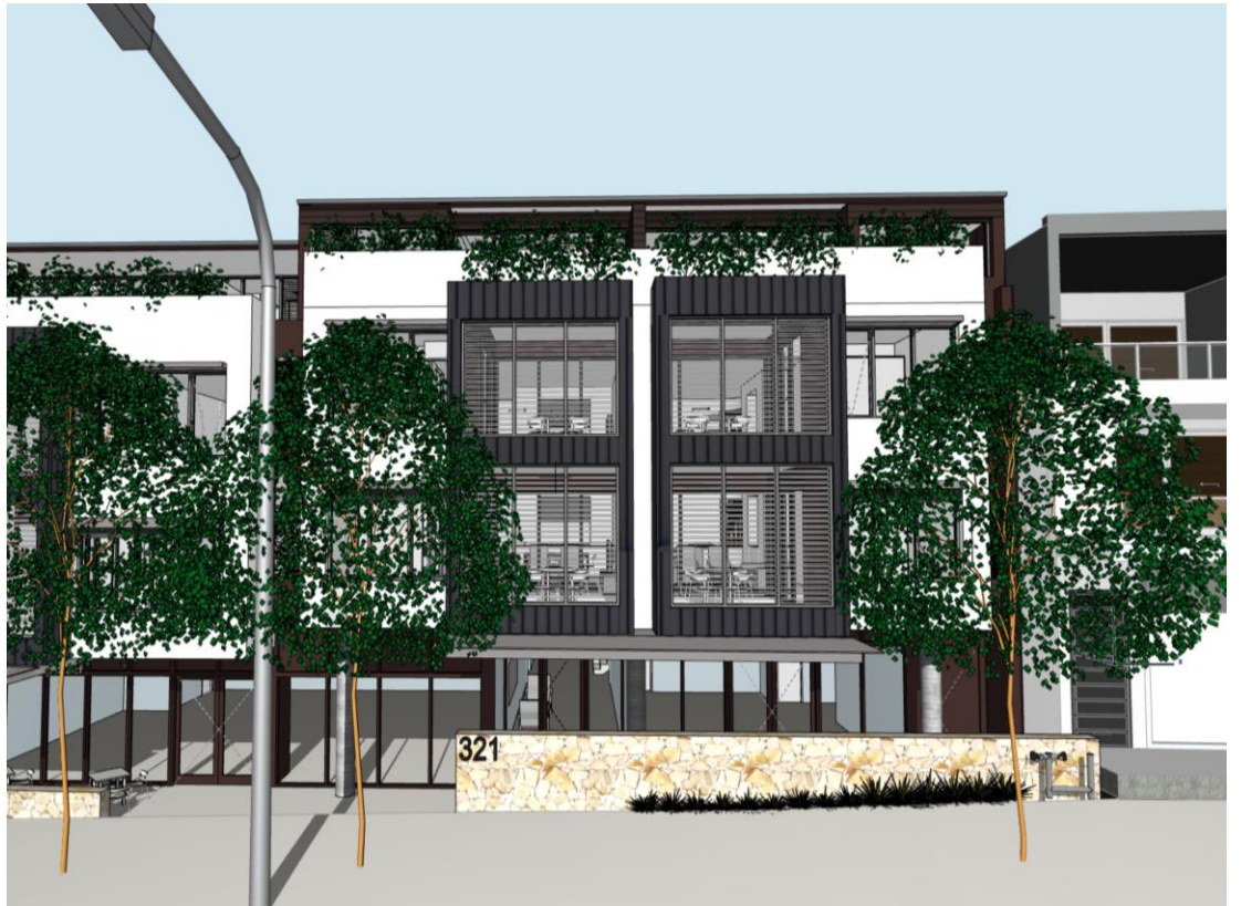
Figure 19: View of Dark grey standing seam cladding on balcony projections.
