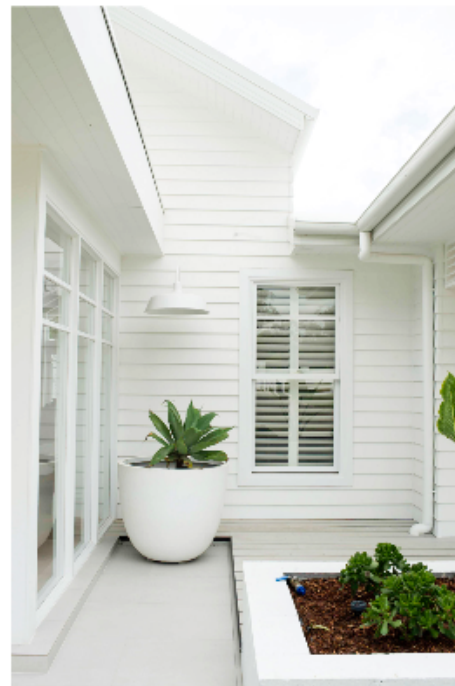
WEATHERBOARD CLADDING
