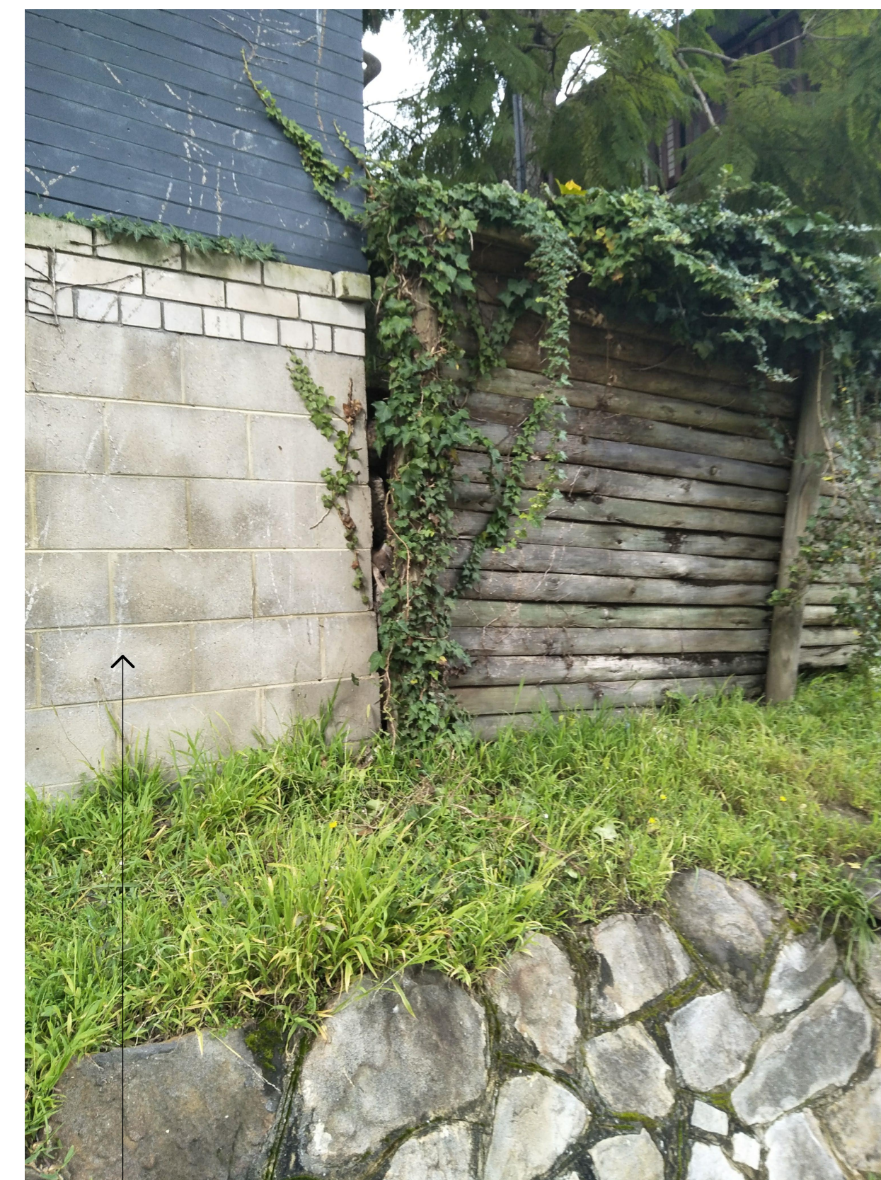
EXISTING TIMBER RETAINING WALL TO BE REPLACED WITH NEW CONCRETE SLEEPER RETAINING WALL TO STRUCTURAL ENGINEER DETAILS
