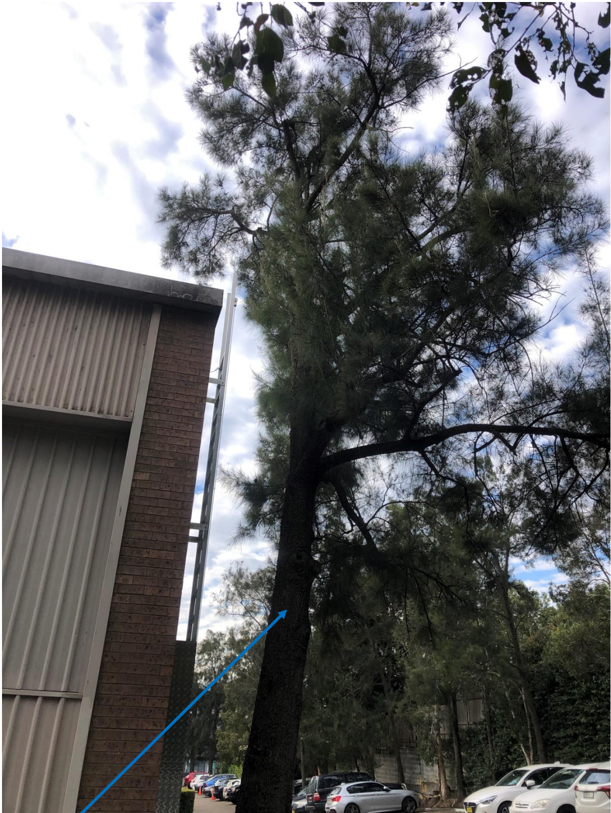
Tree 80 – one-sided canopy
