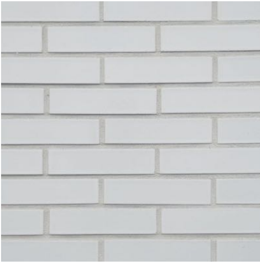
Face brickwork - dwelling additions
