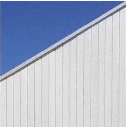
Timber cladding - dwelling additions
