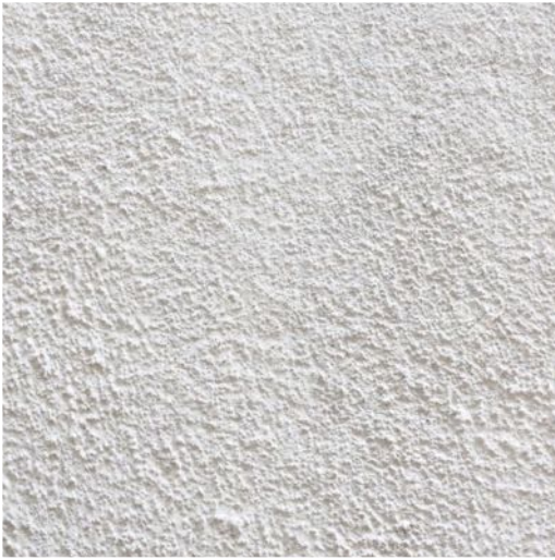
Brick - rendered finish - existing dwelling
