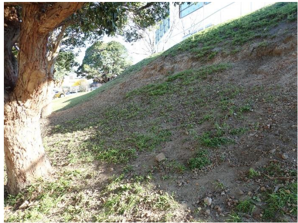
Figure 9 – Exposed clay, crushed sandstone and brick in erosion scour on eastern side of mound.
