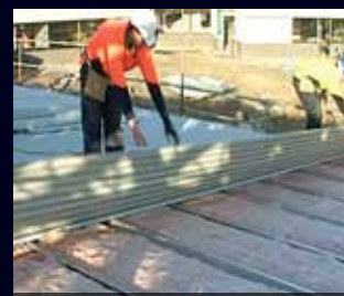
Roof sheet is then tacked in place
