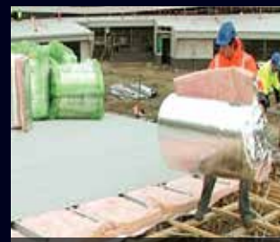
Insulation rolls are "man-handled"
