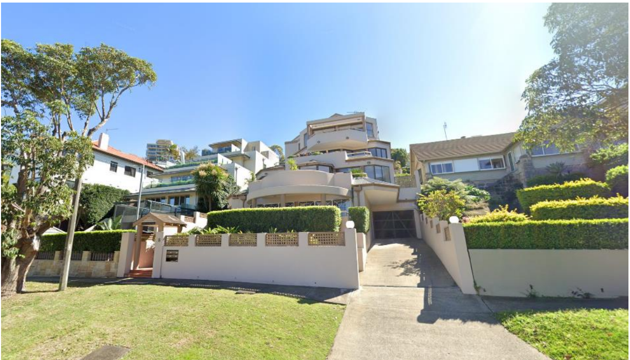
Figure 11: Development downslope of the subject site (northern side of Clifford Ave)
