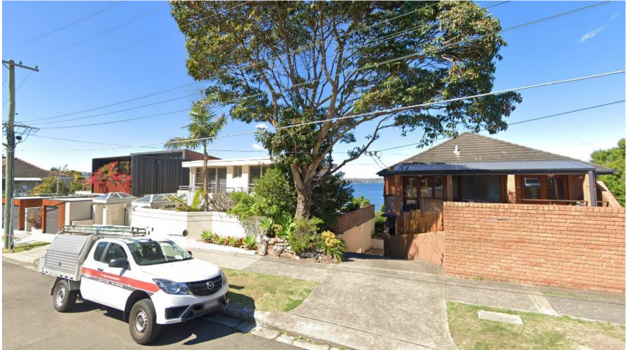
Figure 6: Development to the east of the subject property on Fairlight Street
