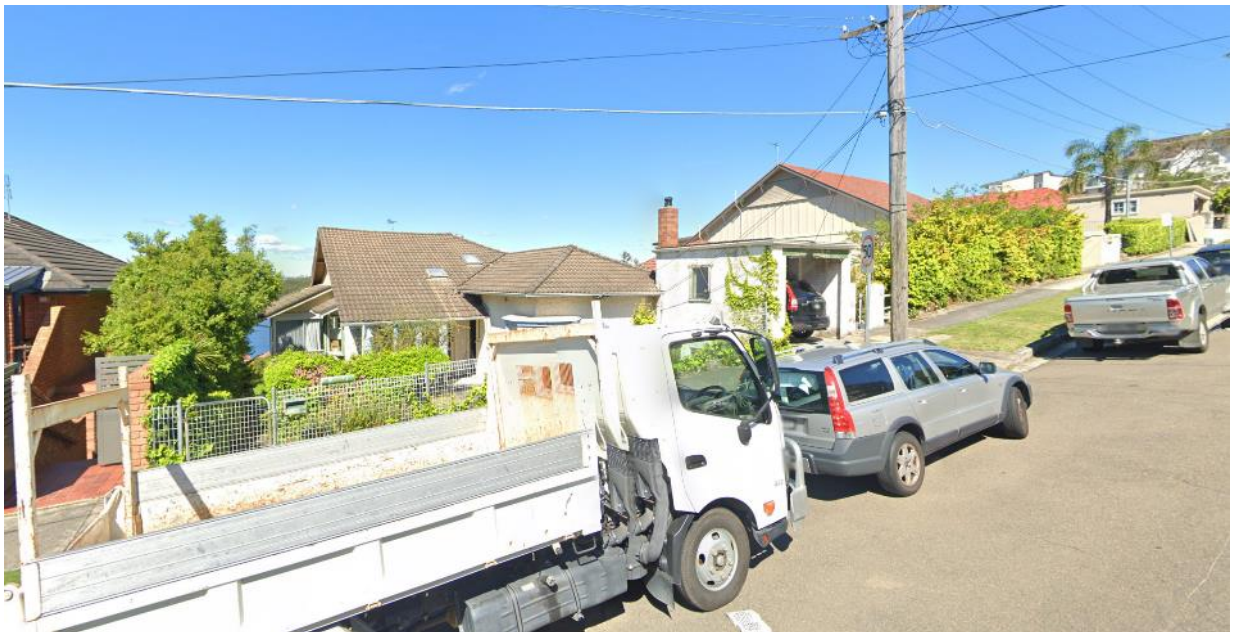
Figure 3: Subject property as viewed from Fairlight Street (east)
