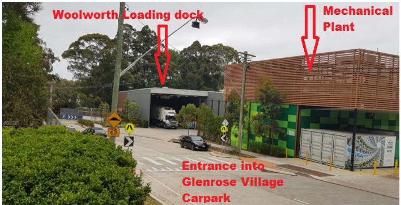
Figure 3 - Surrounding Environment - Glenrose Village (Woolworth loading dock and car park entrance)
