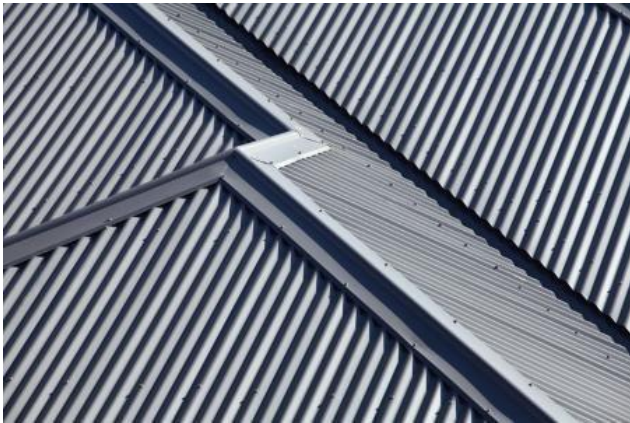
Denotes Sheet Metal Roofing (Typical). Owner To Decide Type & Colour
