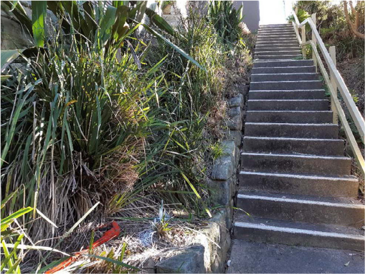
Comms in garden along stairs
