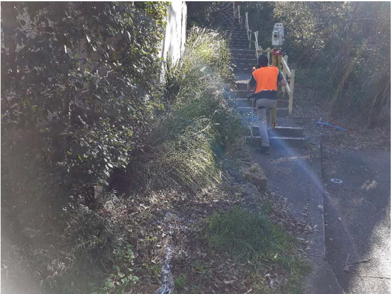
Comms running up garden
