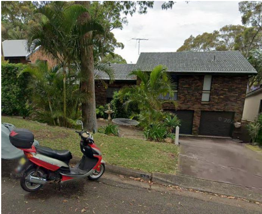
FIGURE 2: Adjacent property, 29 Utingu Place, Bayview 2 Source Google Maps.
