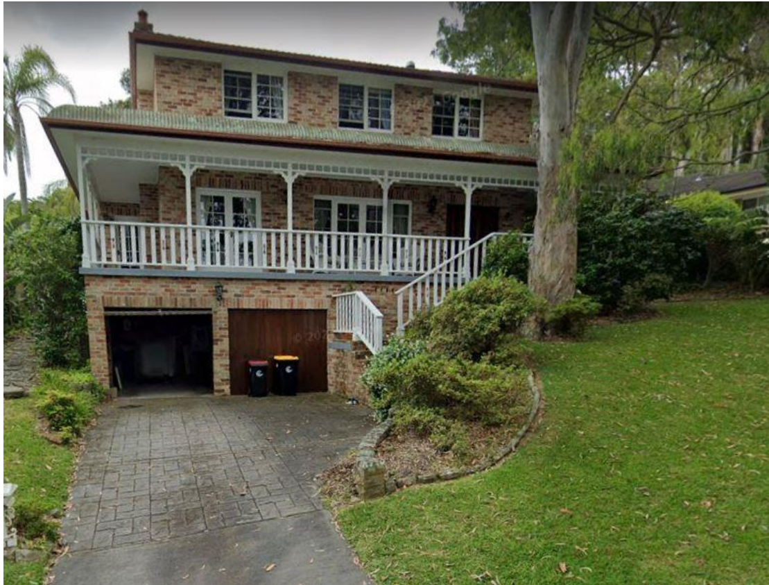
FIGURE 3: Adjacent property, 1 Utingu Place, Bayview 3 Source Google Maps.
