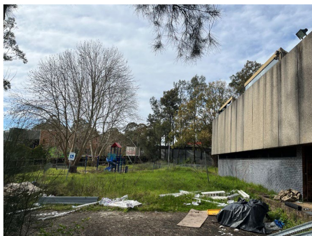
Figure 7: View of the site from the walkway (Prior to demolition)
