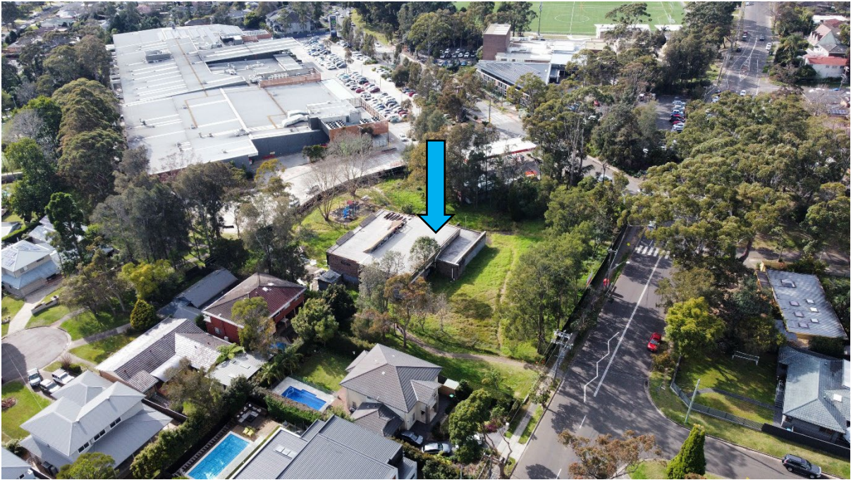
Figure 2: The site looking to the north-east (Prior to demolition)
