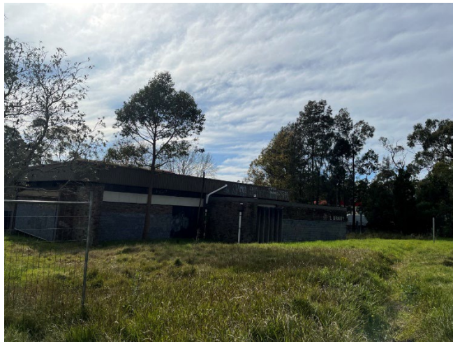
Figure 5: Building from Lockwood Avenue side (Prior to demolition)
