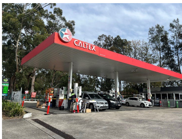
Figure 12: Petrol station to adjoining the site to the east
