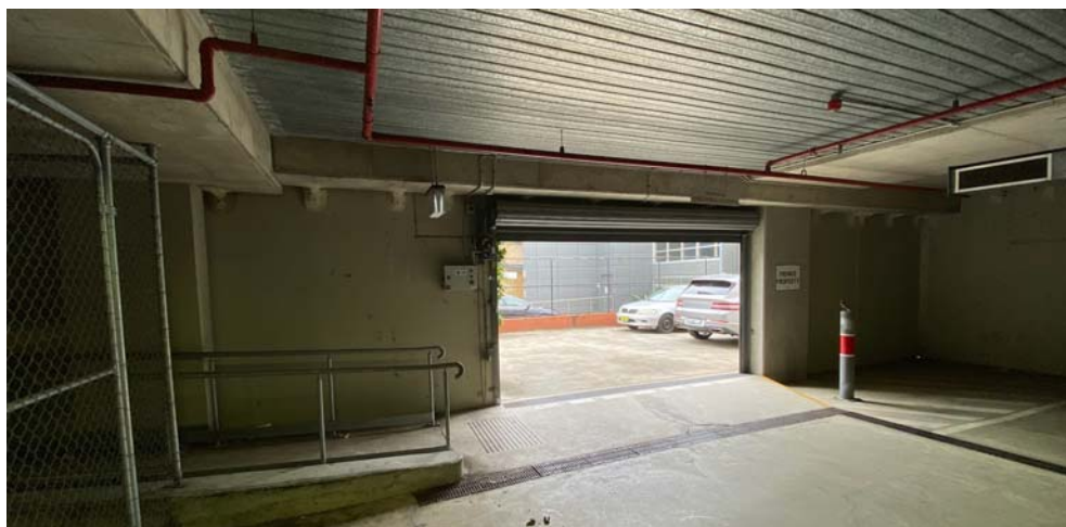
Photograph of the access opening to 1749 Pittwater Road
