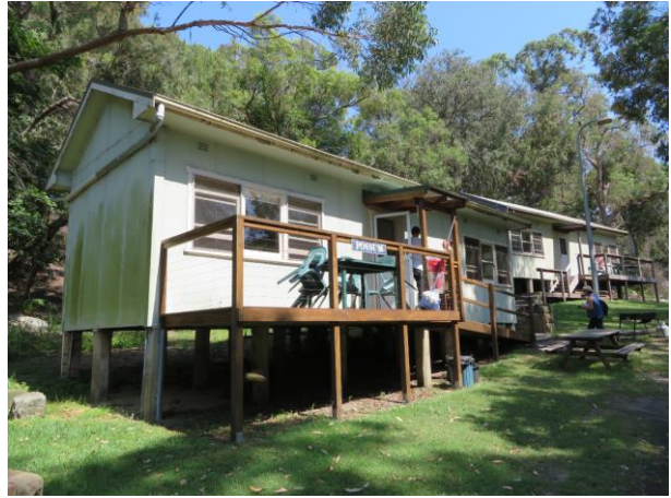
Figure 20 – Cabin 7, Possum , facing north-west.
