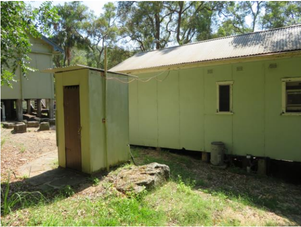
Figure 21 – Rear of Cabin 7, Possum , facing north-west, including outhouse.
