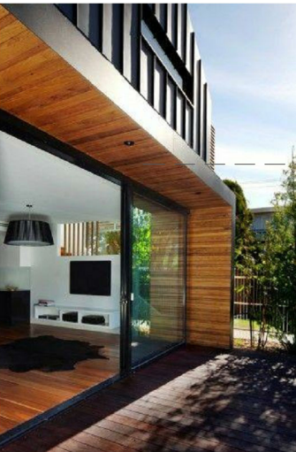
timber soffits - shiplap clad - natural finish
