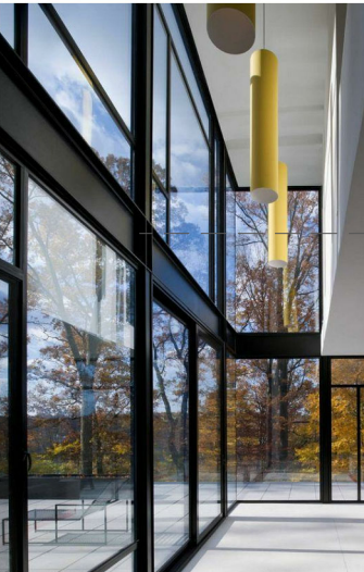
exposed structural steel + window hoods - painted 'matt black'
