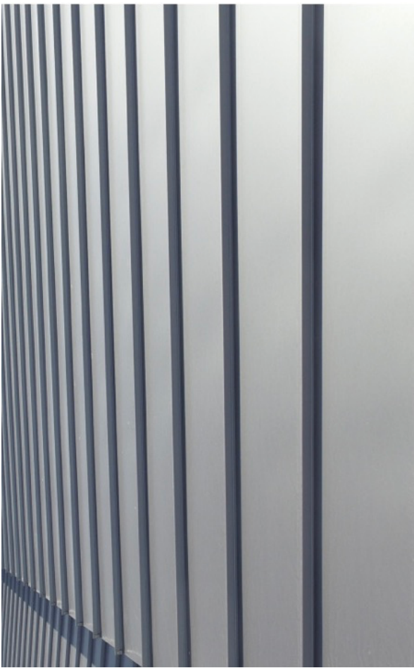
04 _ MID GREY COLOURED TRAY ROOFING
