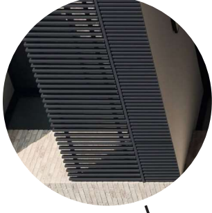
BLACK STEEL HANDRAIL
