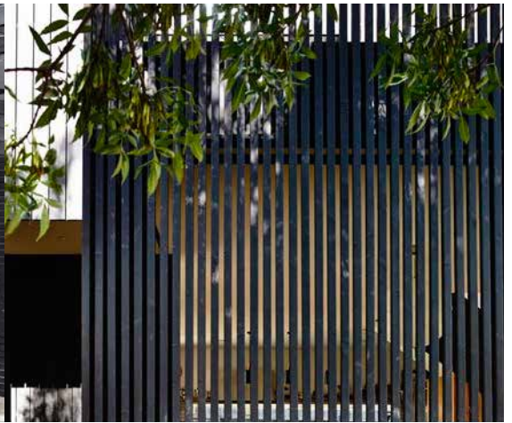
BLACK STAINED TIMBER BATTENS - 50% OPEN
