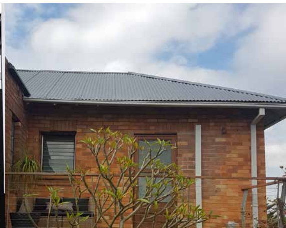
MID GREY METAL ROOF TO MATCH EXISTING
