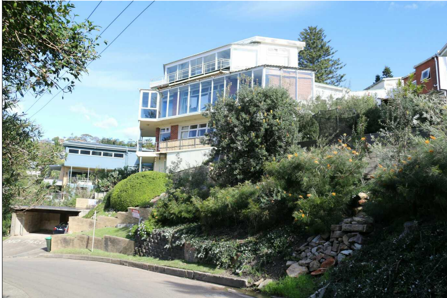
VIEW OF EXISTING BUILDING FROM SURF ROAD
