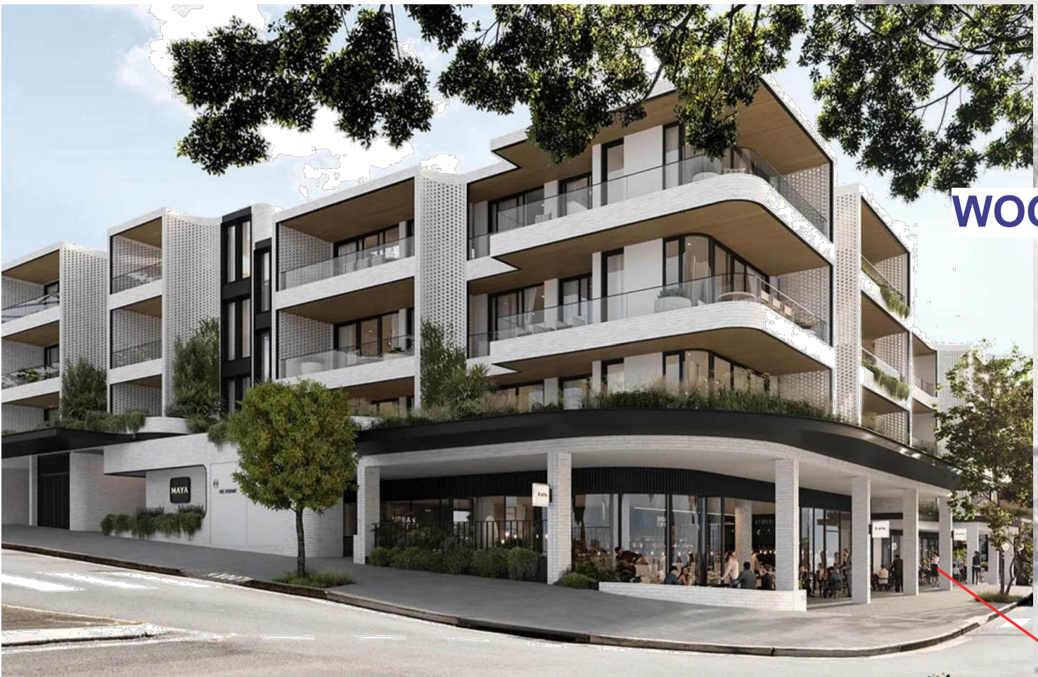
9 BUNGAN STREET STOREY BUILDING
