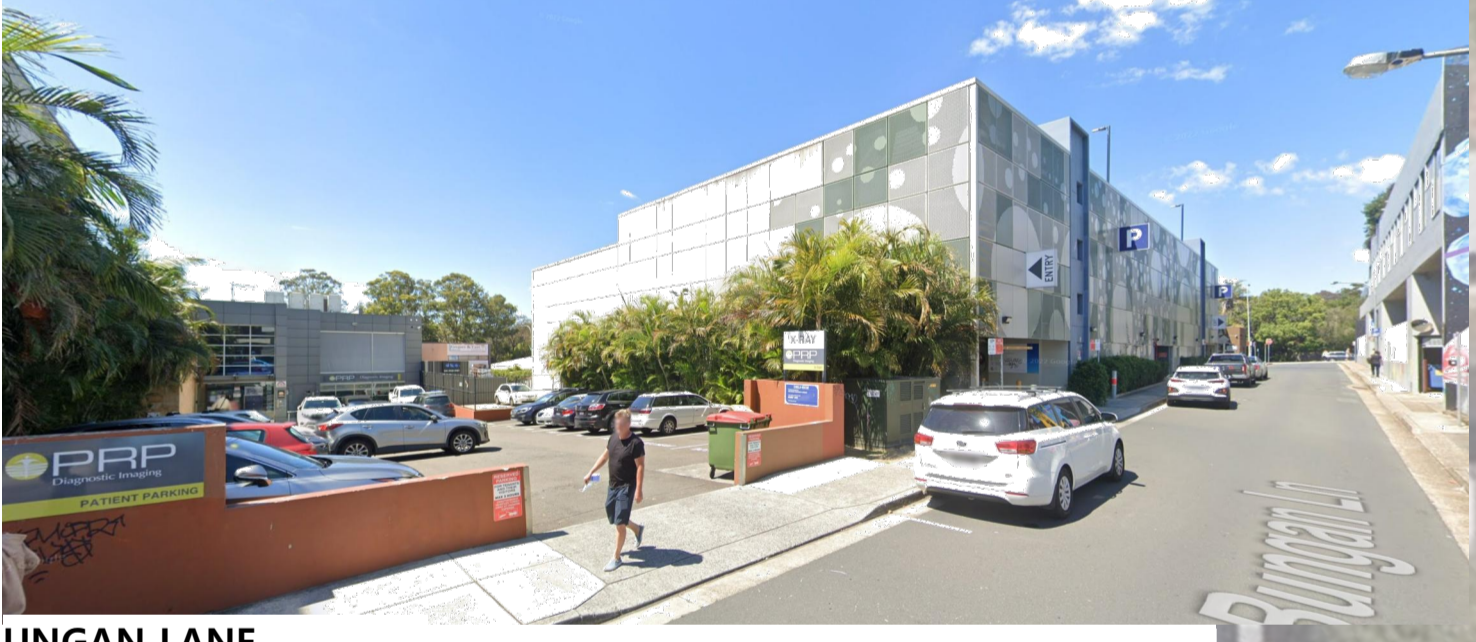
BUNGAN LANE EXISTING ENTRY TO SITE
