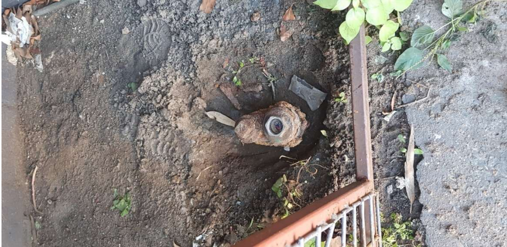
Figure 5 - Valve/pipe believed to be associated with the tank/bowser, located under the stairs in the car park.
