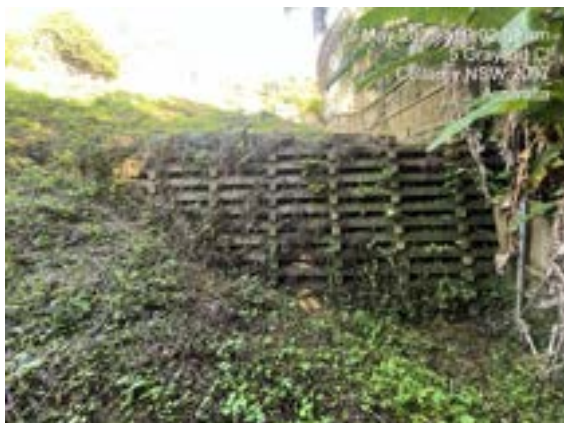
Photo 6: Concrete crib wall in north-eastern corner of the site.
