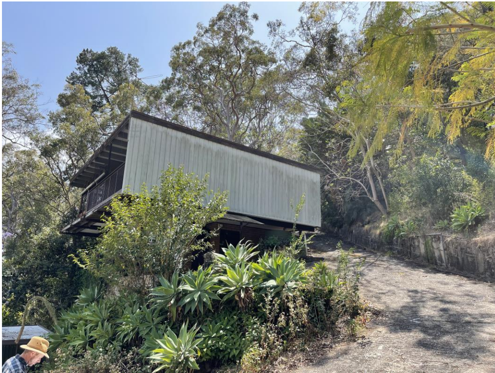
Fig 7: View of the existing dwelling at No 143 Riverview Road, looking north-east
