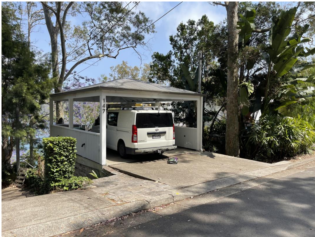
Fig 3: View of the neighbouring carport structure at No 147 Riverview Road, looking north west
