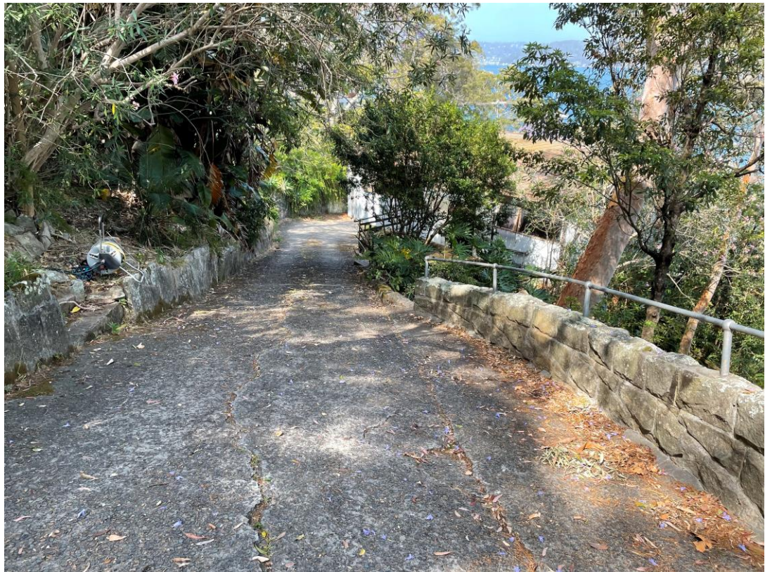
Fig's 4 & 5: Views of the common access driveway to the site, looking south-west
