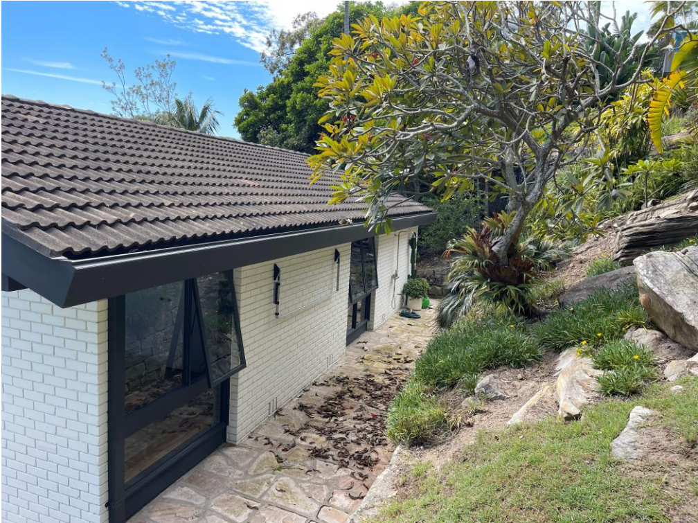
Fig 9: View of the rear elevation of the dwelling, looking east
