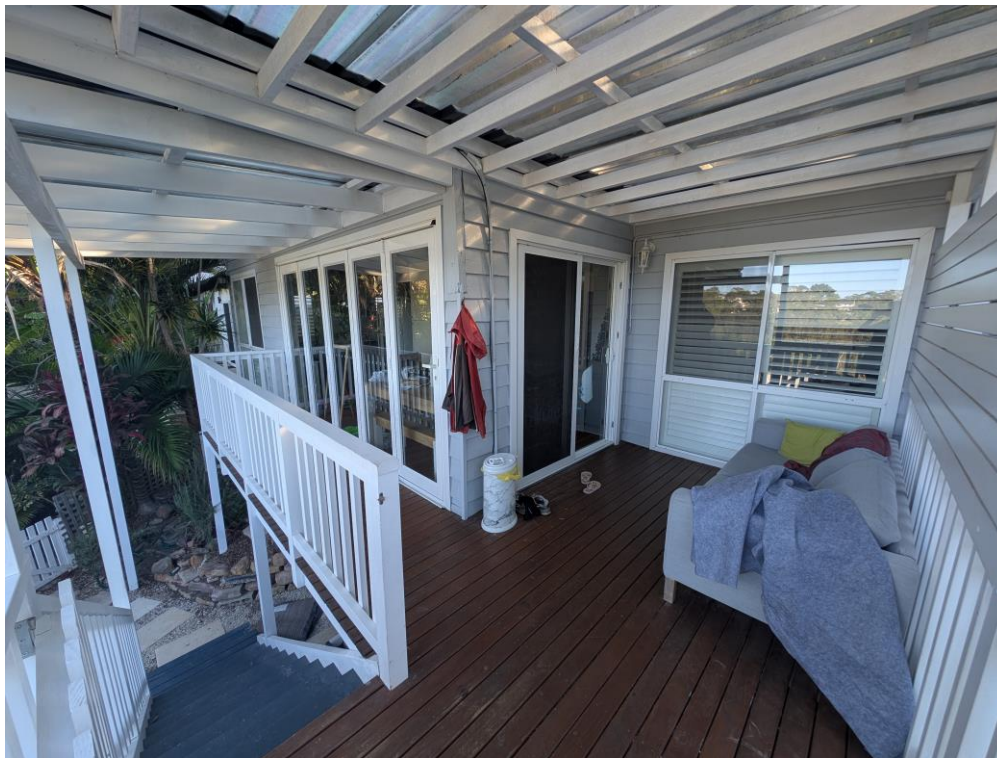
Image 9 – View of existing house entry (ground floor) and covered deck. Stairs are proposed to be internalised by boxing in recessed deck area shown) and accessed from new Lower Ground Floor entry. Existing bi-folds to be retained, deck extended and re-covered with new roof.
