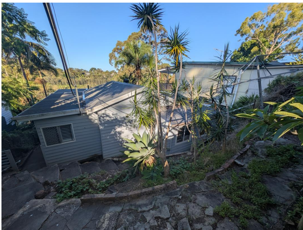
Image 8 – View looking North-East showing existing dwelling and rear garden with existing dilapidated concrete stairs and masonry walls. The proposal seeks to run the existing rear wall of the study across the back of the dwelling to increase internal space as well as carry the existing roof shape (central pitch – flat sides) to the front and back.
