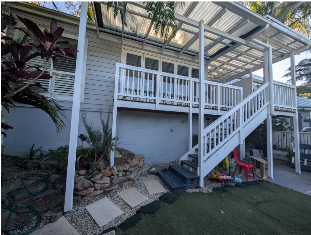
Image 3 – View of front garden area and front house facade within property (partially above existing single garage) in need of improvement. Brick wall proposed to be opened to create entry to new Lower Ground Floor area. Deck to be replaced, extended & re-roofed.
