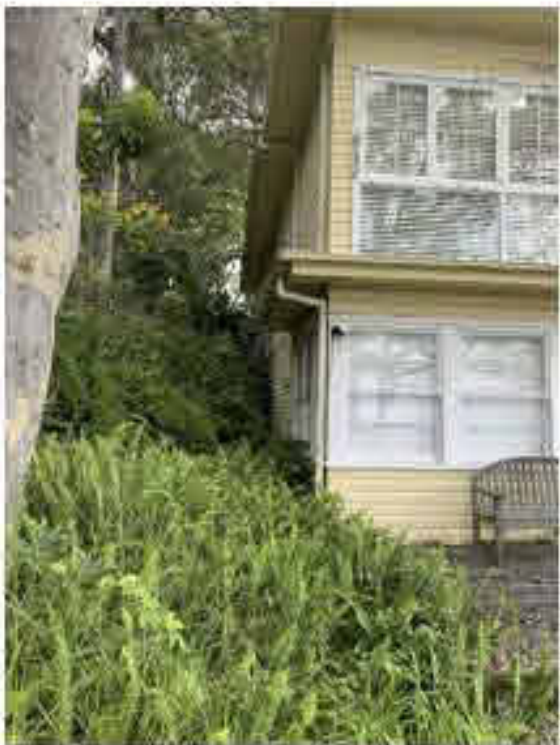
EXTG - REAR OF HOUSE
