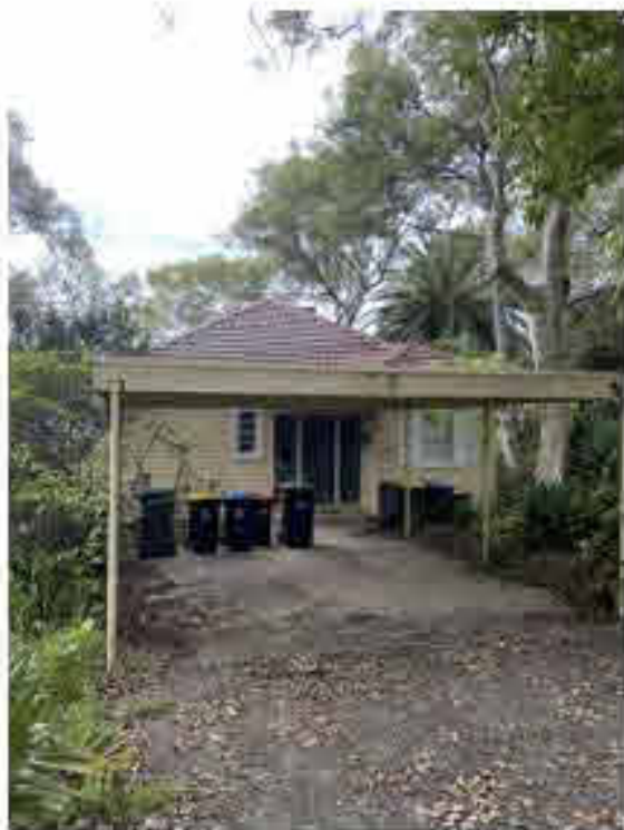
EXTG - FRONT OF HOUSE
