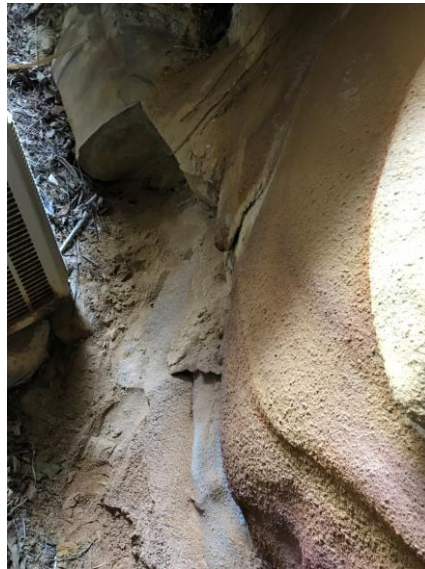
Photograph 10: Accumulation of eroded sandstone to the south of the site structure
