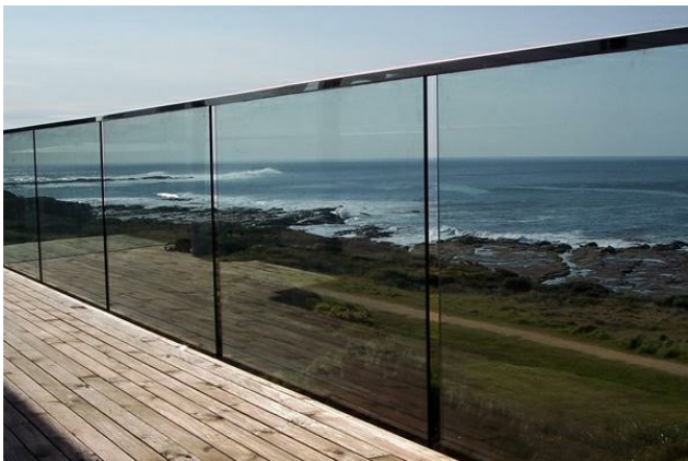
GLASS BALUSTERS WITH TOP RAILING
