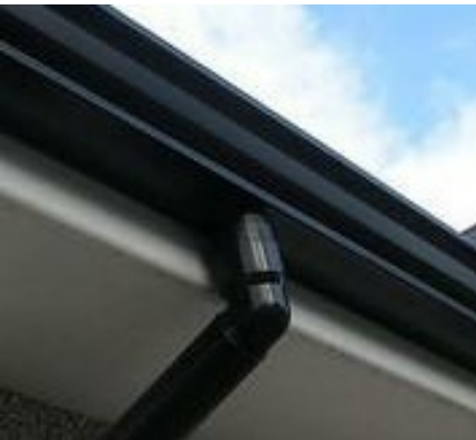
DARK/ BLACK FASCIAS, GUTTERS AND DOWNPIPES
