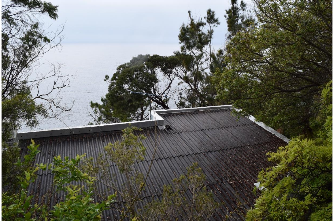
Figure 29: The cement fibre sheet roofing of the subject site, looking east.
