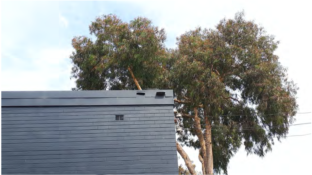
Photo 4: Extent of canopy overhanging building.
