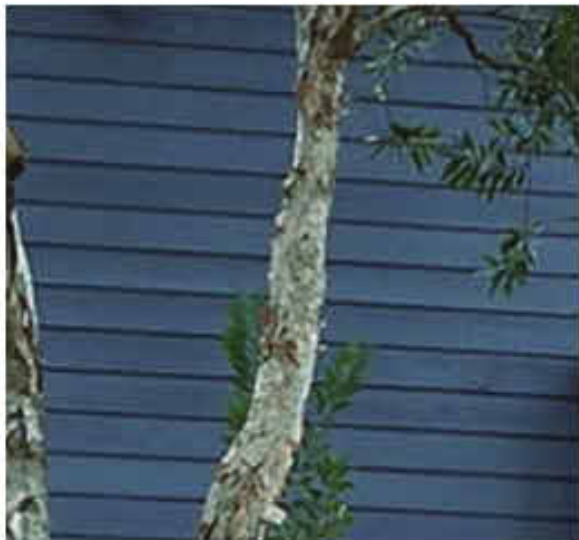
New cladding to match existing in both profile and colour
