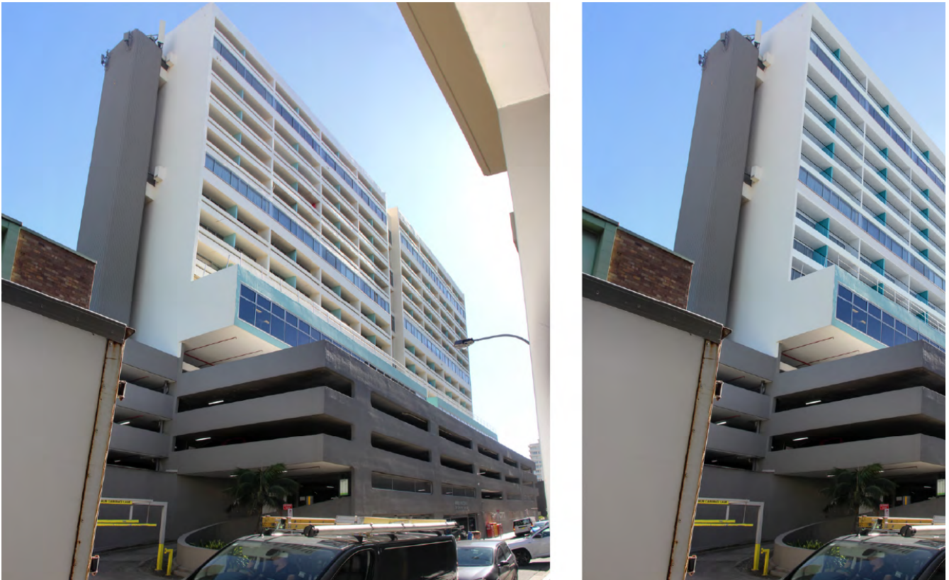
Figure 1. Existing concrete balustrades (left) and proposed glass balustrades (right) (Source: Urbaine Architecture).
